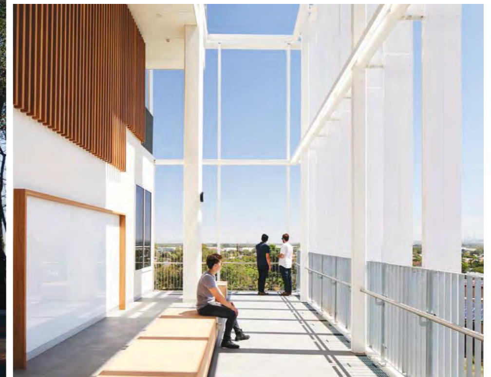
Australian Catholic University Mercy Building
