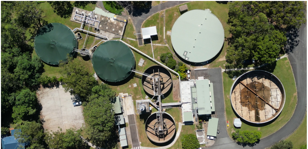
Capalaba Water Treatment Plant, next to Leslie Harrison Dam.
