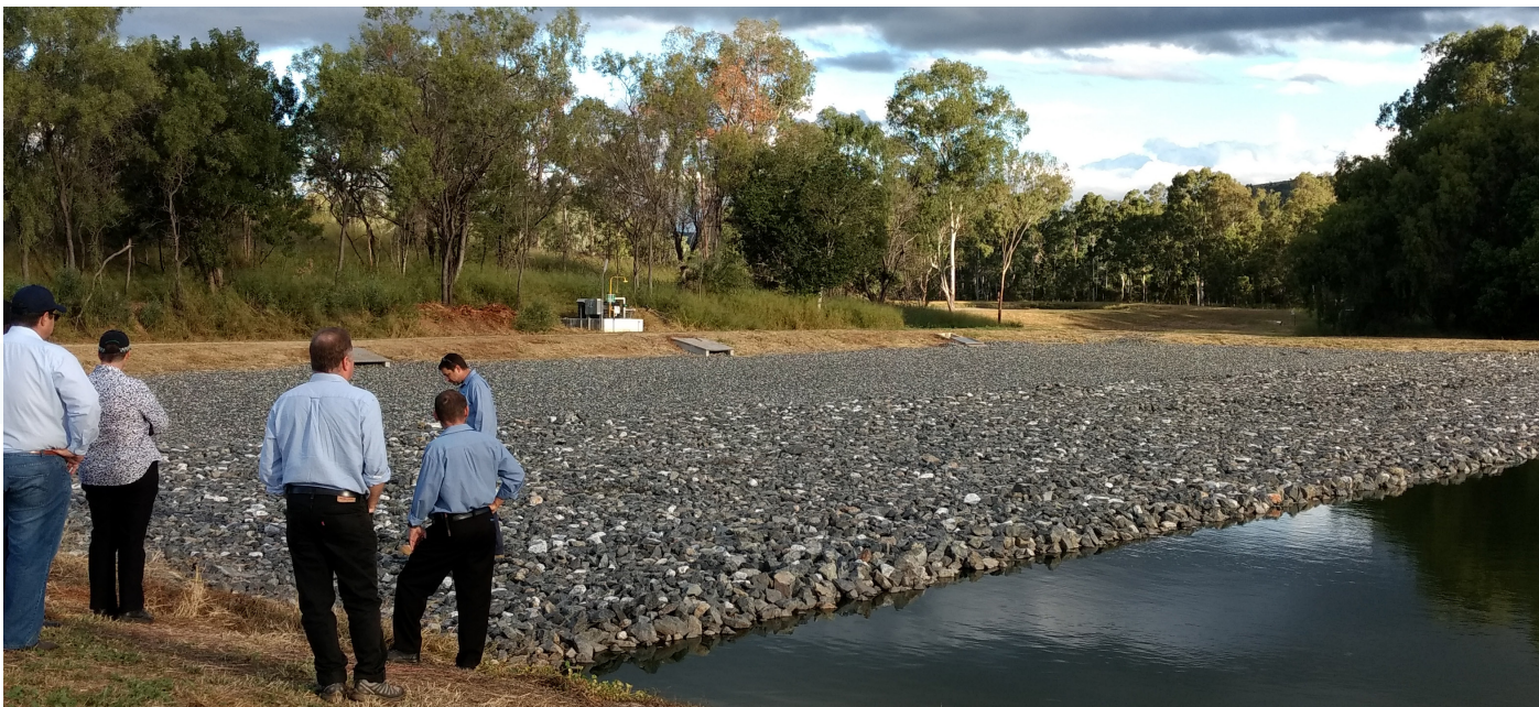
Rock Filter at Gaynah Waste Water Treatment Plant, May 2017
